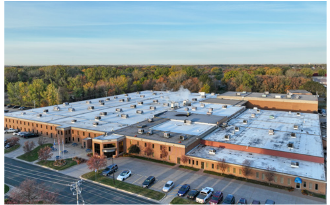
The Wilson Tool headquarters in Minnesota is one of seven manufacturing sites worldwide.
